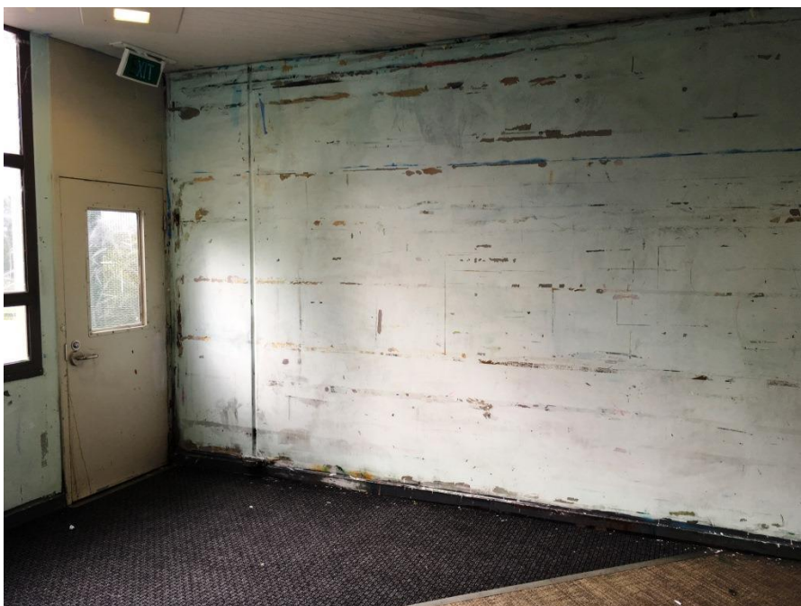
Photo 2: Inside Te Marama Unit
