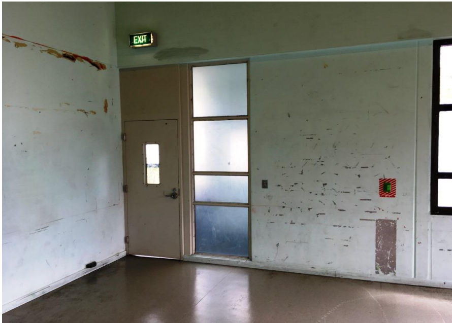
Photo 1: Inside Te Marama Unit
