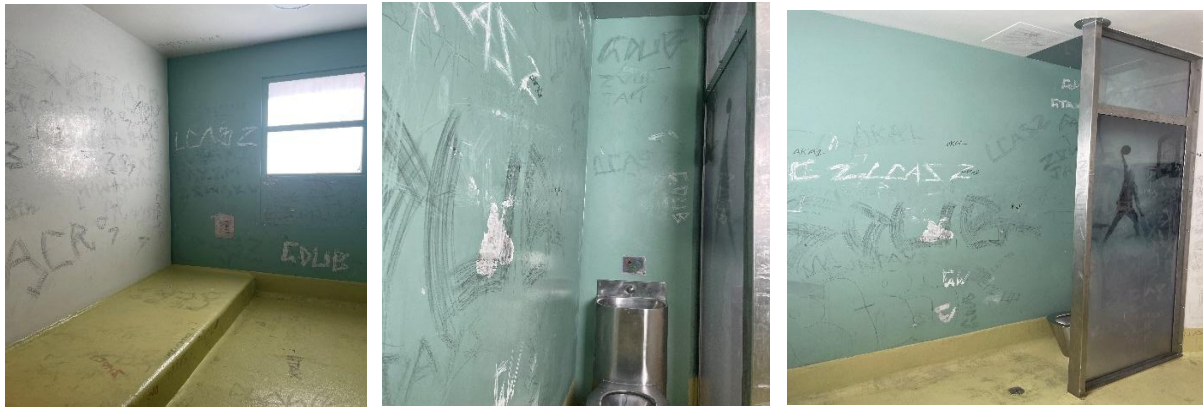
(Bedroom and toilet area in Secure Care)
